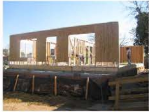
1218 Pine Street: Construction
